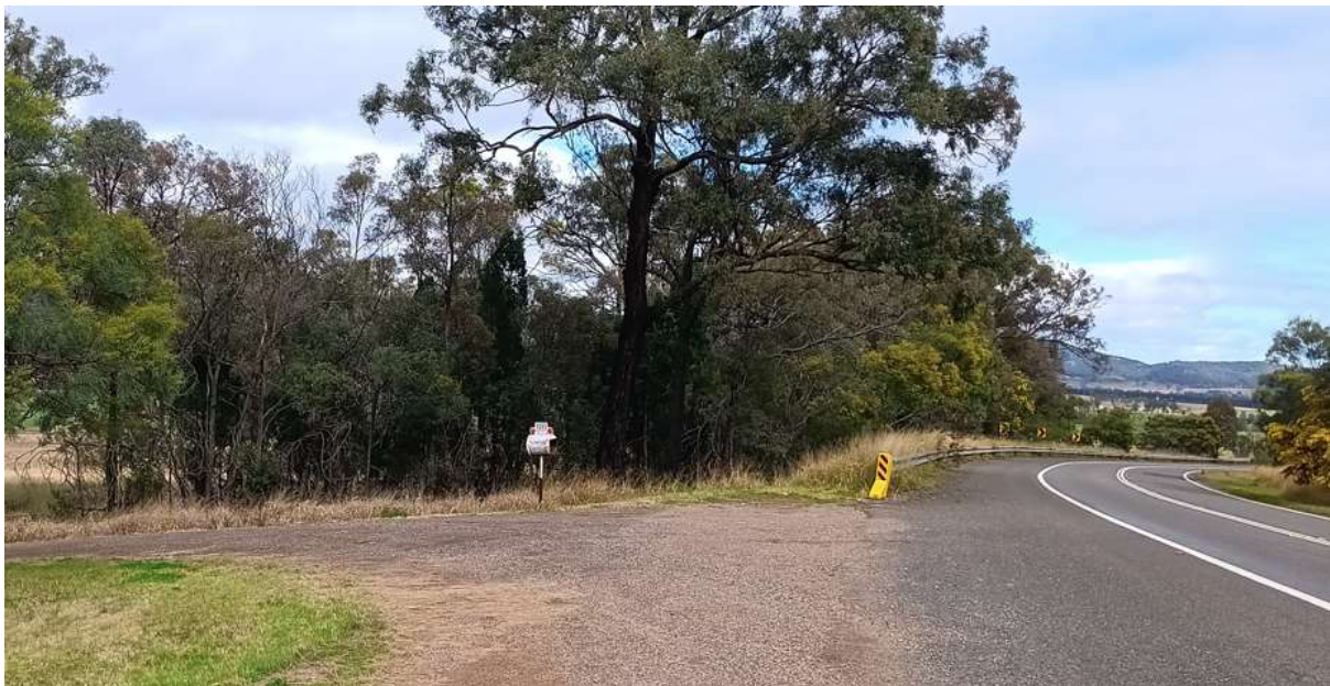
Figure 5 – Looking west towards Sandy Hollow
